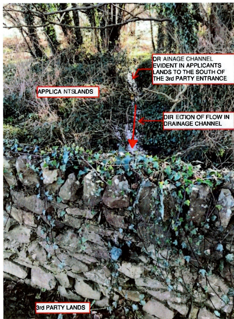
Figure 1 Image of the existing “eastern drainage channel” within the applicants lands
